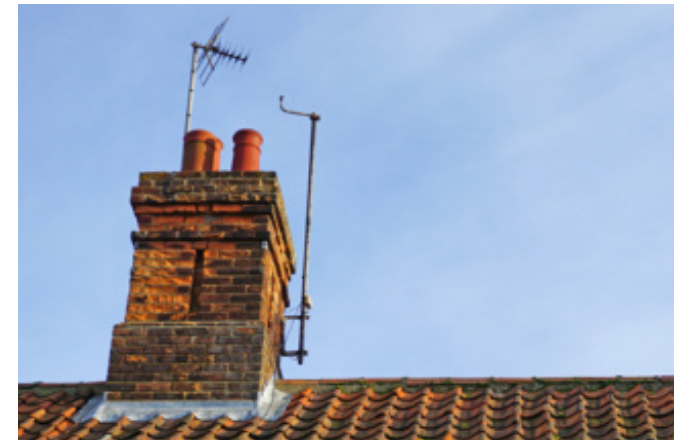
Eroding brickwork on a chimney
