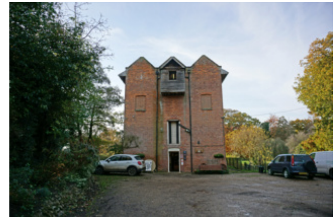
Letheringsett Mill, east elevation
