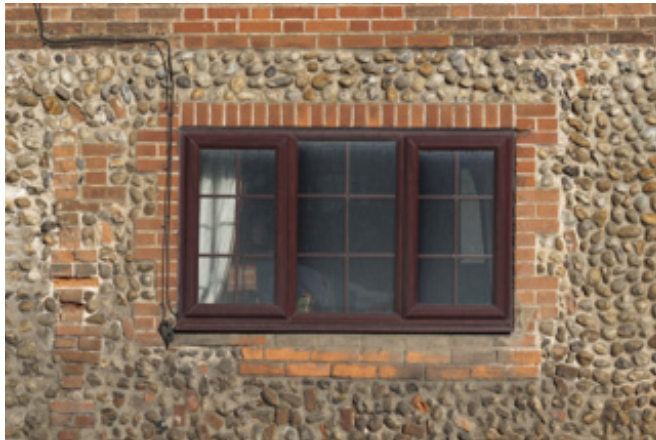
Inappropriate uPVC window
