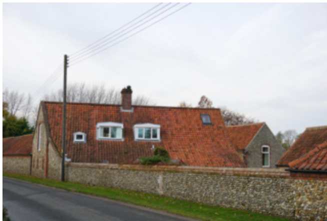
Converted barn at Home Farm
