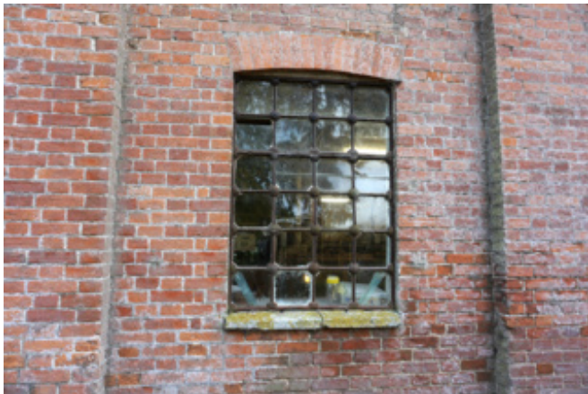
Rusting and bowed window on the mill
