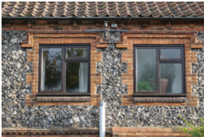
Though timber, the replacement windows do not have the original pattern of glazing bars and openings and the dark stained finish is not as appropriate as a light coloured paint. The image also shows a pale coloured plastic vent pipe
