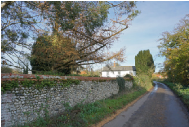
Flint and brick wall on Riverside Road
