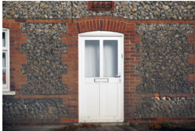
Inappropriate uPVC door
