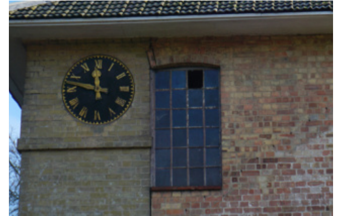
Rusting window frame with glass pane missing
