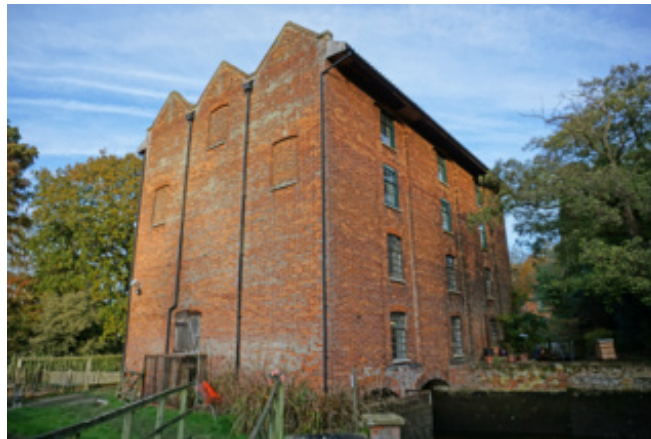
Letheringsett Mill, west and south elevations
