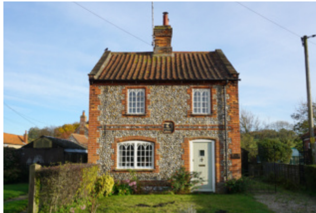
Cottage in Little Thornage with more decorative detail than the older vernacular cottages
