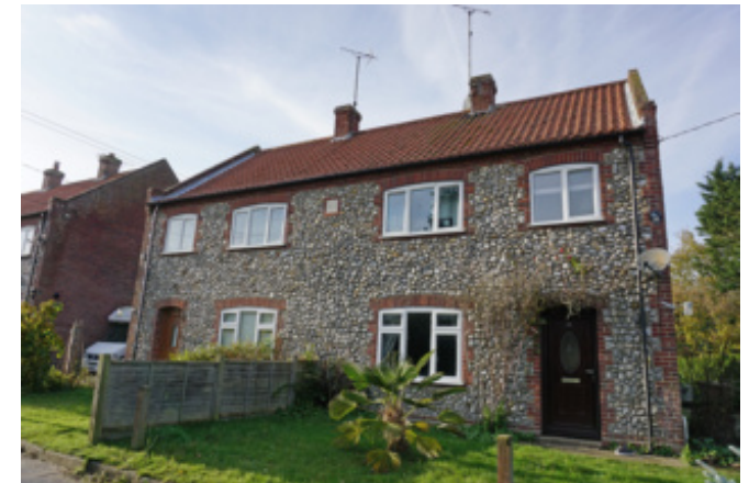
Modern cottages on Riverside Road
